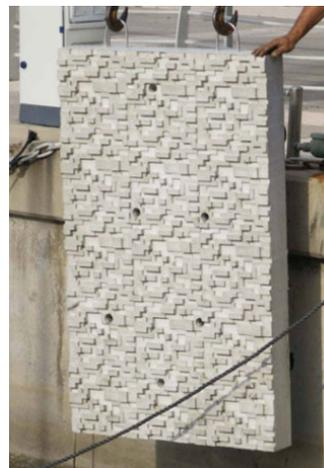
ECONcrete® panels in a seawall
