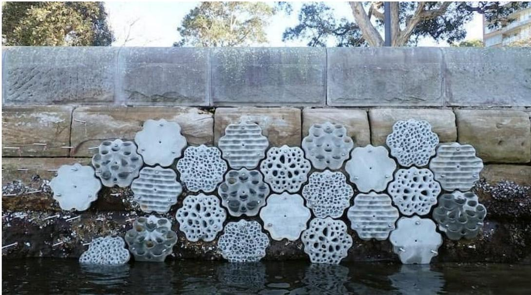
Figure 12 Living Seawalls at Sydney Harbours. [Source:<https://www.sustainabilityhackers.com/living-seawalls-to-bring-new-life-to-rushcutters-bay/>]
