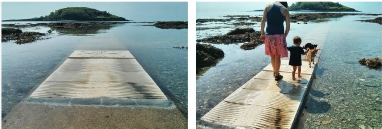
*Figure 15 Eco-enhanced stormwater outfall at Hannafore beach*
