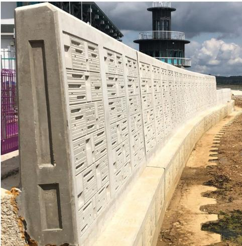
Figure 5 Technique 4 Cast-in textured, grooved and creviced concrete surfaces
