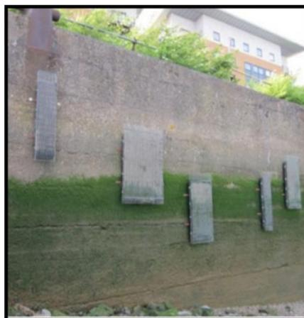
Figure 8 Technique 7 – Bolt on green wall modules
