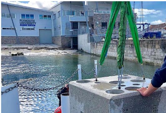
Figure 11 BIOBLOCK being lifted into place [Source: <https://www.plymouth.ac.uk/news/bioblocks-show-how-coastal-designs-could-benefit-marine-life>]
