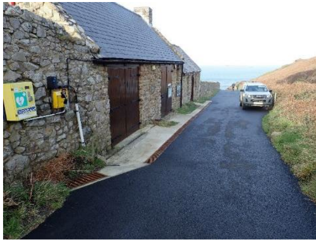
Figure 5.2 Martins Haven improved access road and drainage at Fisherman's Cottage
