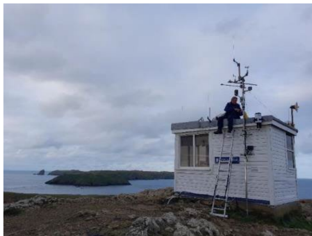
Figure 5.4 Weather station maintenance work.
